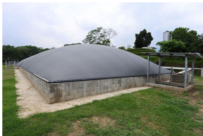
Slika 13. Lagunski digester (Anonymous 1, 2019).
