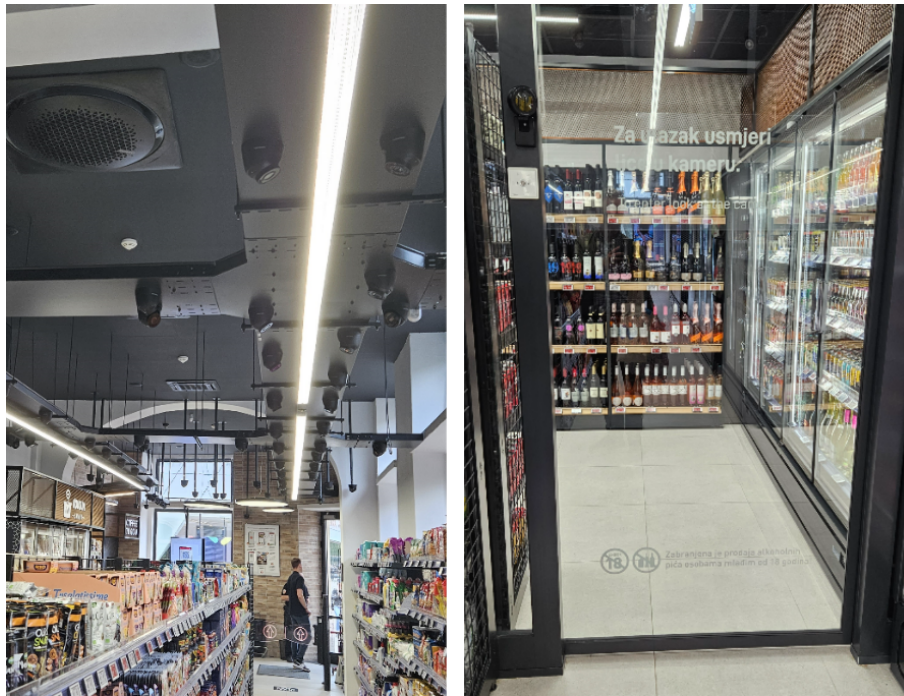
Figure 1.2: Access control system (right) in a smart store (left) preventing minors from entering the section containing age-restricted products (i.e., alcoholic beverages).
