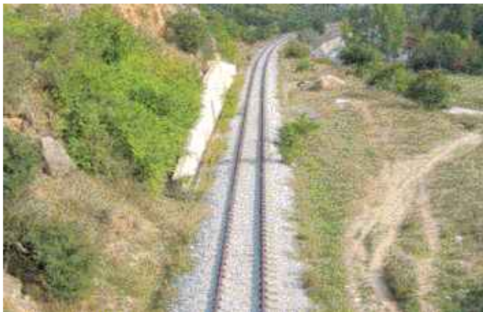
Figure 7 Rehabilitated section Kumanovo – Beljakovci
