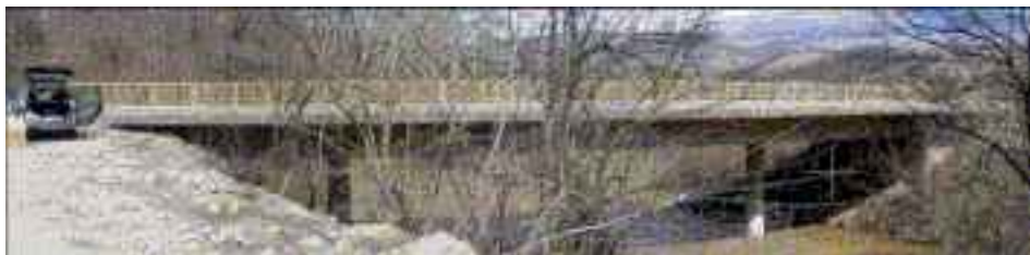
Figure 1 Upstream view of the existing bridge
