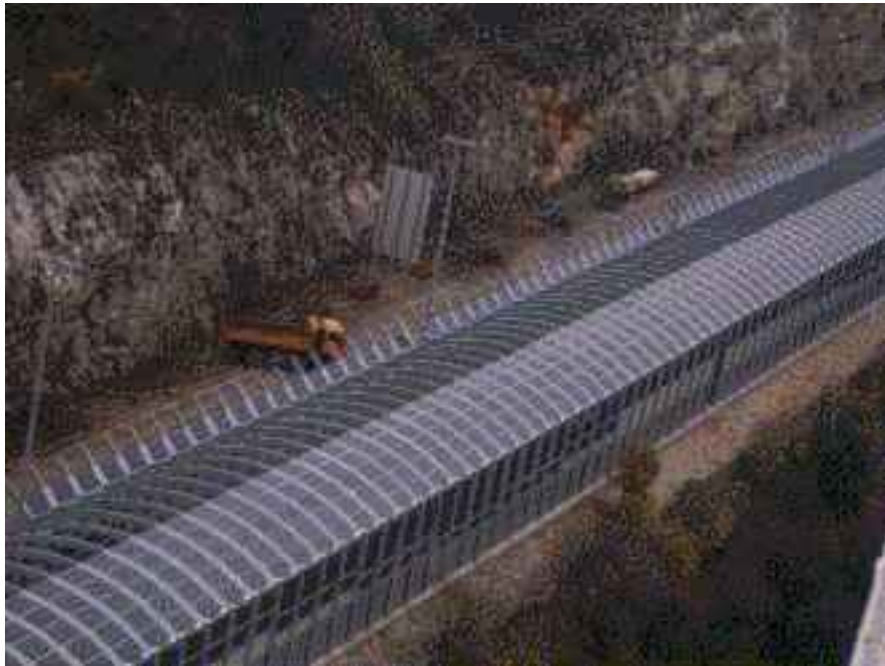
Figure 3 View towards the solar noise protection wall from the south.
