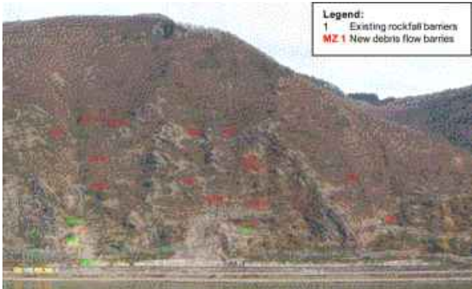
Figure 7 Installation complete with old rock fall barriers and new installed debris flow barriers. (Source of Fig. 7: Institute of Environmental Planning, Dr. Kübler GmbH).
