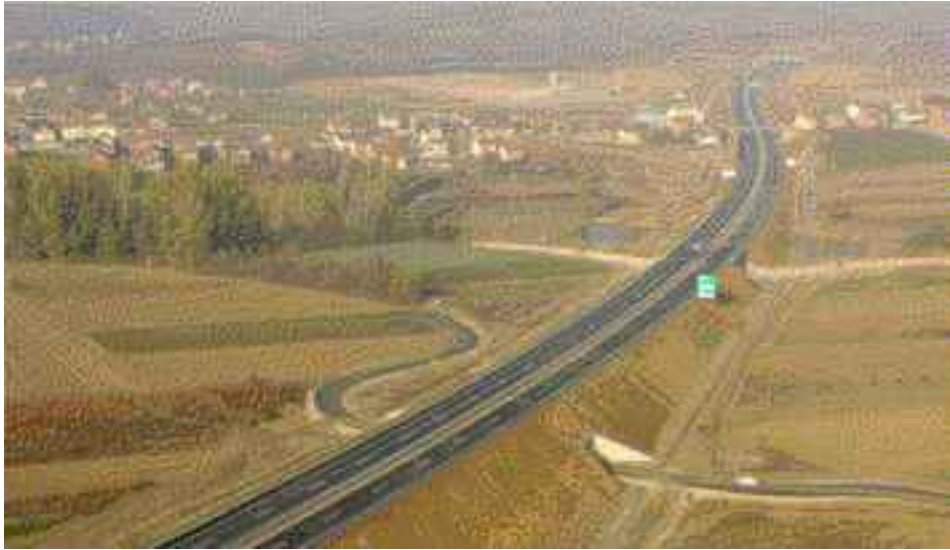
Figure 11 Completed motorway on the large embankment part.
