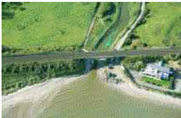
Figure 2 Aerial view of UB65 bridge, looking upstream
