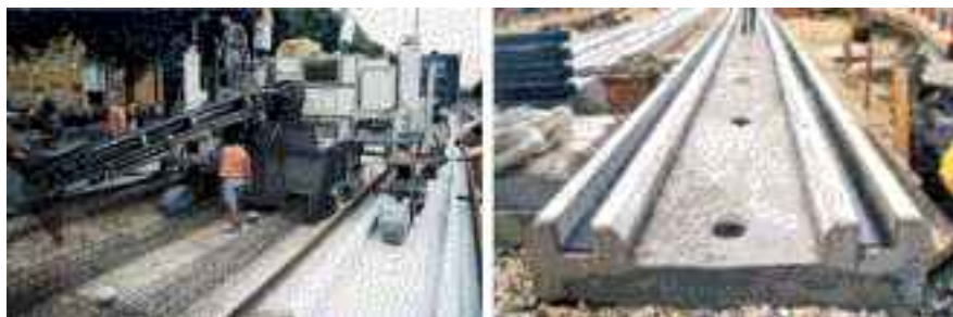
Figure 6 INFUNDO/EDILON system
