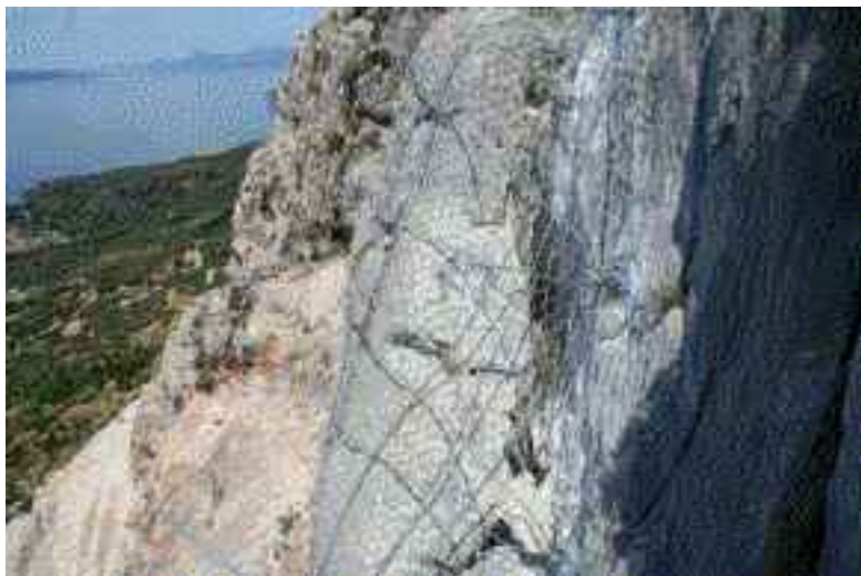
Figure 7 Retaining unstable boulders
