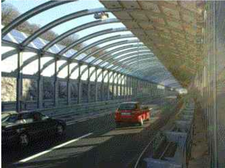
Figure 4 Constructed integral system – view from inside.
