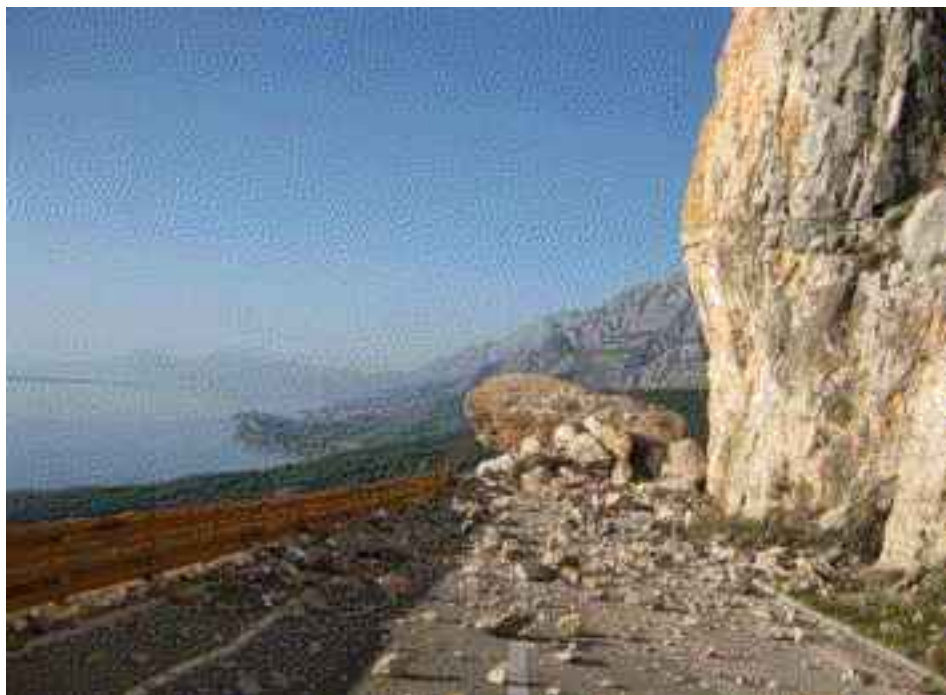
Figure 1 The rockfall on the D512 state road
