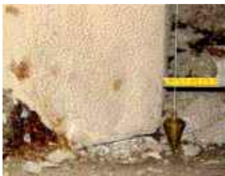
Figure 2 Vertical impairment and deviation of bearings
