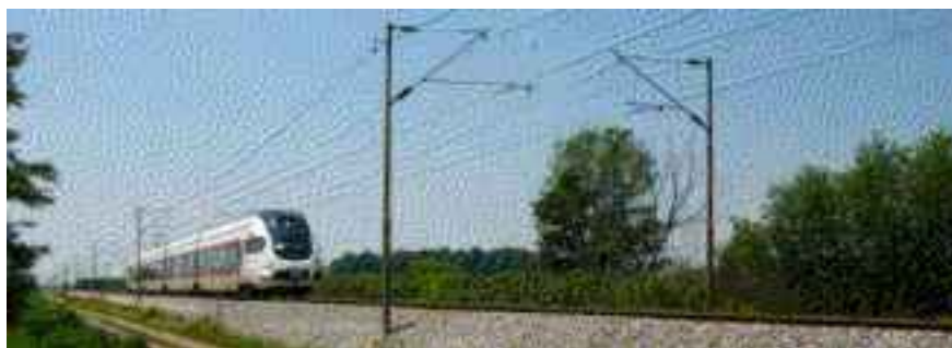
Figure 1 Test section on Vrpolje – Ivankovo railway line with tested EMV
