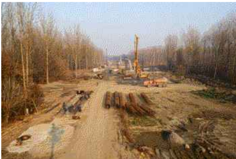
Figure 7 Construction site on the Drava River Bridge
