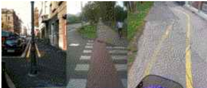
Figure 3 Deficiencies and inconsistencies in the existing bike paths and lanes which should be removed
