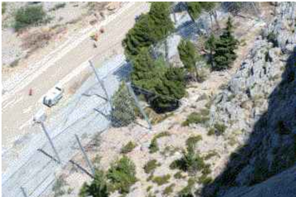
Figure 6 Constructed barriers Retaining unstable boulders
