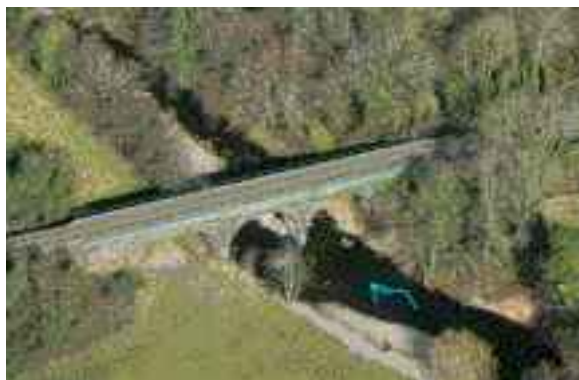
Figure 4 Aerial view of UB18 bridge, looking upstream.
