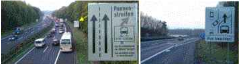
Figure 6 Road signs to indicate that regular service buses are permitted to use the emergency lane (text on the left: emergency lane ... Mon.-Fri. 6:00-9:00 a.m. ... only for public buses to exit Dornach (text at the bottom in Czech) text on the right: Watch for buses!)
