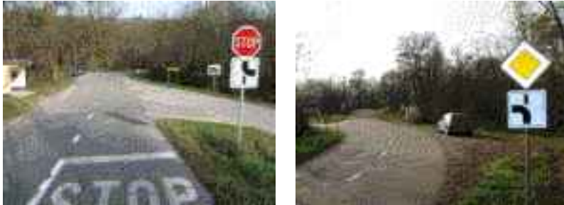
Figure 6 Misleading information: signs vs. road markings (horizontal line gives the illusion of right-of-way driving strait ahead)
