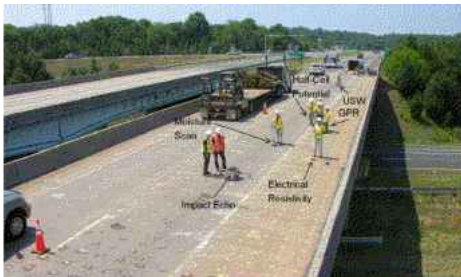
Figure 4 NDE survey of a bridge in Virginia.
