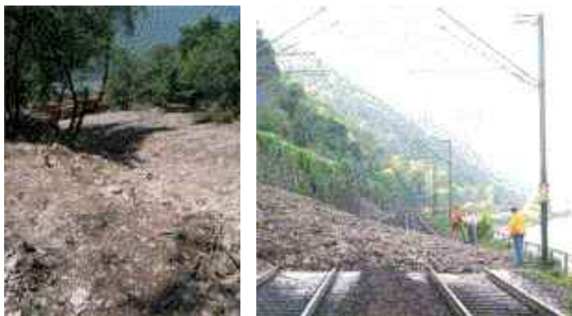
Figure 1 Steep slope with loose material above the river Rhine (left) and material deposited at the railway line after the event in July 2008 (right).
