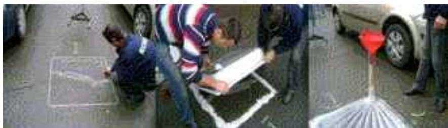
Figure 4 Surface marking; Sealing material application; Field device
