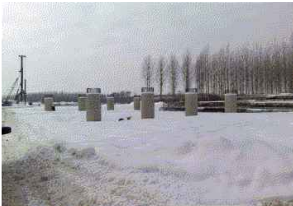
Figure 6 Construction works on the Drava River Bridge
