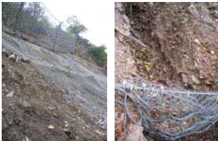
Figure 6 Slope stabilisation for the loose deposited material (left) and small debris brake at a gully to reduce the flow energy level (right).
