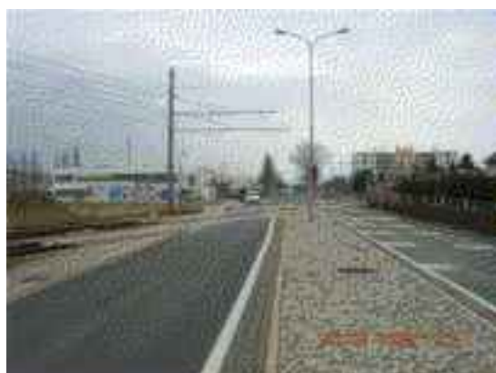
Figure 8 Two-track light rail changing sides of a road (Badener Bahn at LB17, Traiskirchen, Austria). Photo: T.Brezina.
