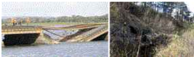
Figure 1 Left: Collapse of Malahide Viaduct on the Belfast–Dublin rail line (August 20th 2009); right: Rainfall induced slope failure at Merano, Italy (April 2010)
