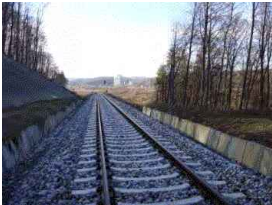
Figure 4 Special track of cement factory Našicecement
