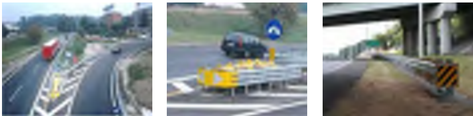
Figure 6 Safe barrier systems with proper ends
