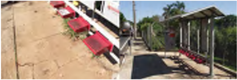
Figure 3 Examples of regularized sidewalks with curbside cutouts for easy access to people with reduced mobility, however, with the absence of elevated curbside to facilitate boarding of wheelchair users
