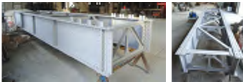
Figure 7 Bridge in process of rehabilitation
