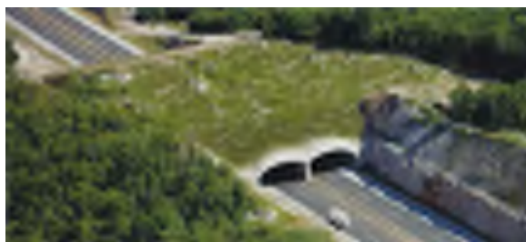
Figure 1 Wildlife crossing on Croatian motorway [2]
