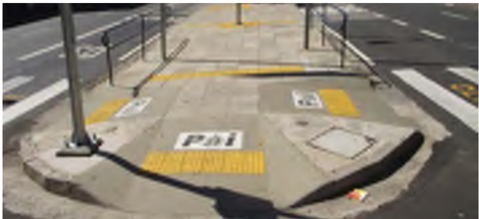
Figure 8 Ramps to facilitate access of persons with disabilities or reduced mobility
