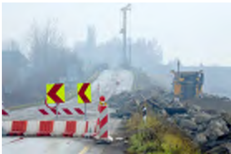
Figure 5 The construction site on Southern bypass of Osijek: overpass “Bosutsko”
