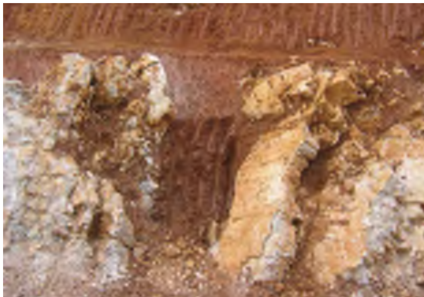
Figure 5 Subsoil shaft along fault
