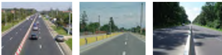
Figure 7 Safe median barriers
