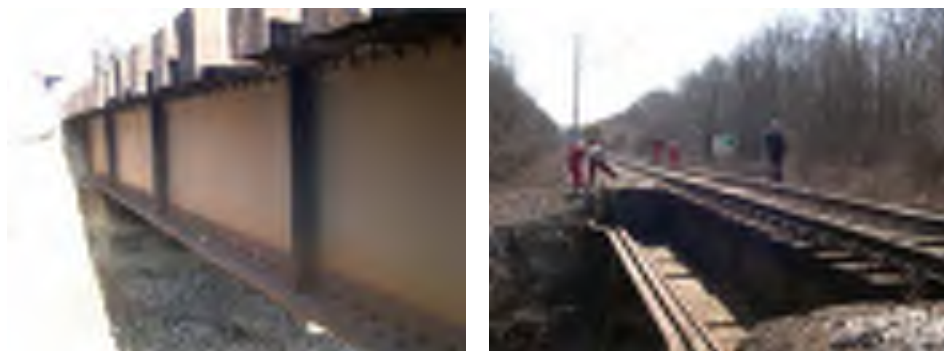
Figure 1 Location of Buna bridge
