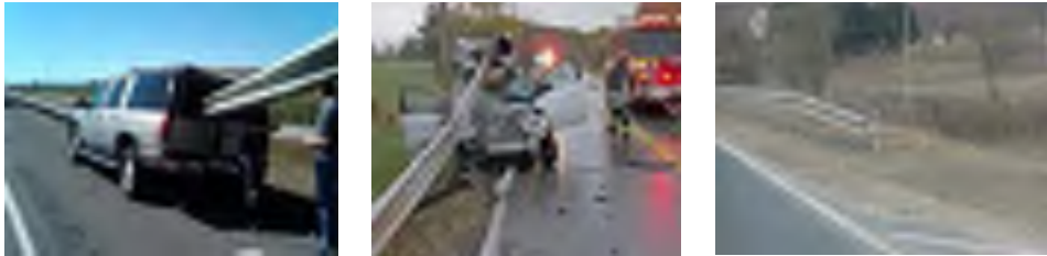
Figure 5 Unsafe barrier systems
