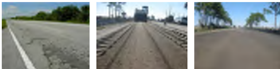
Figure 4 Martin County jobsite in Florida : before, during and after
