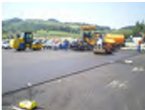
a) b) Figure 2 Construction of test field with PMMA/ATH composite dust in wearing course in 2009 (a.) and the same test field in 2013 (b).
