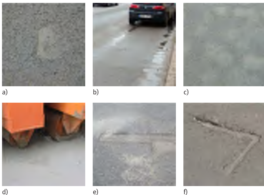
Figure 1 Examples of permanent deformation observe in pavements of special objects: a) port; b) parking lot; c) parking apron of aircraft; d) e) f) industrial area
