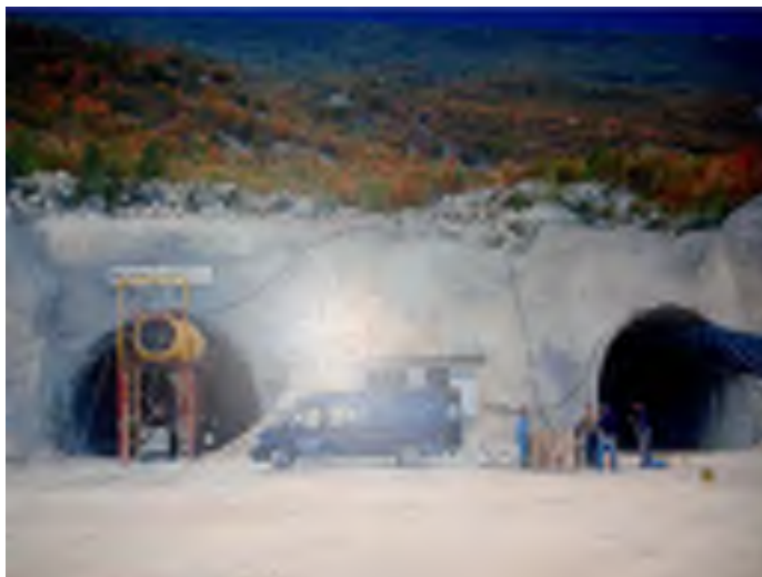
Figure 3 The north portal of the main and service tunnel tube
