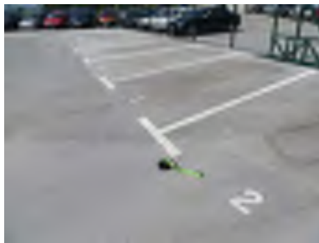
a) b) Figure 2 Construction of test field with PMMA/ATH composite dust in wearing course in 2009 (a.) and the same test field in 2013 (b).
