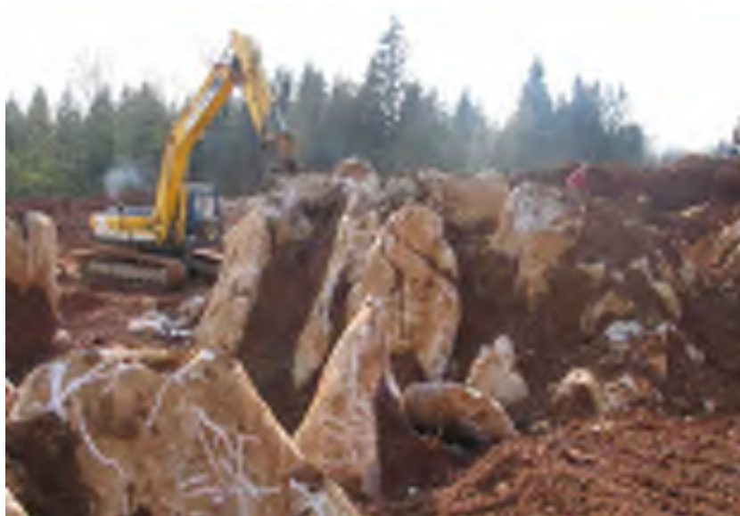
Figure 1 Uncovering of subsoil stone forest
