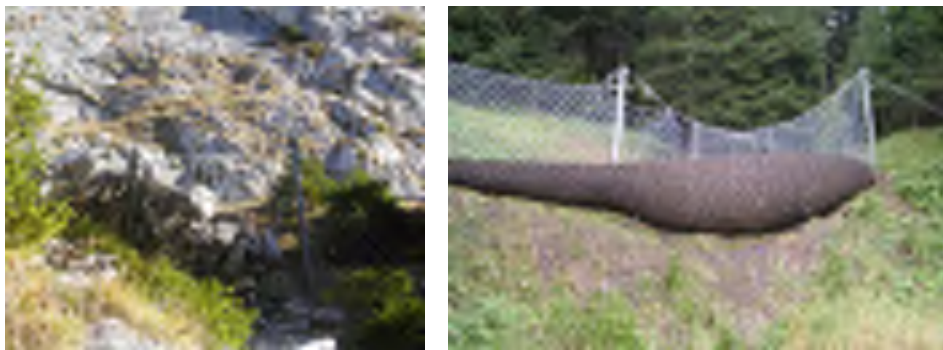
Figure 1 Snow net barrier loaded with rockfall (left), rockfall barrier loaded with a shallow landslide (right)
