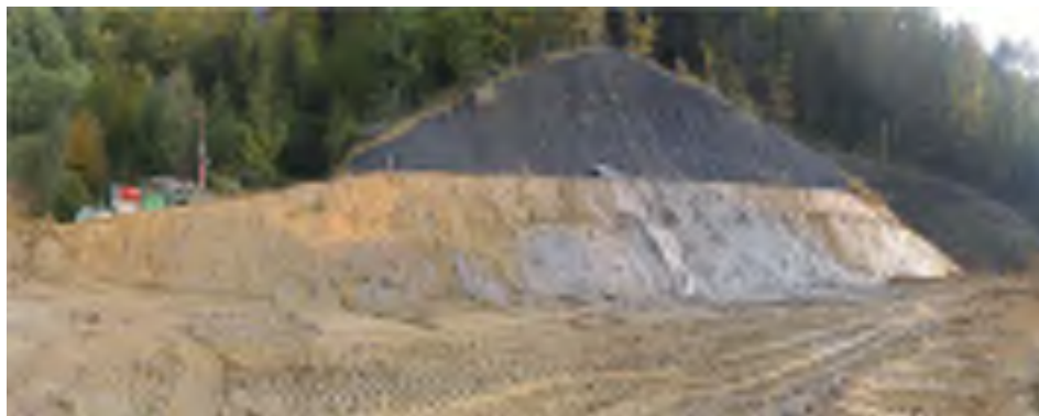
Figure 1 Gornji Macelj 4 cut during construction.
