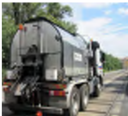
Figure 3 Resurfacing TRAMWAY (PRAGUE 2012)
