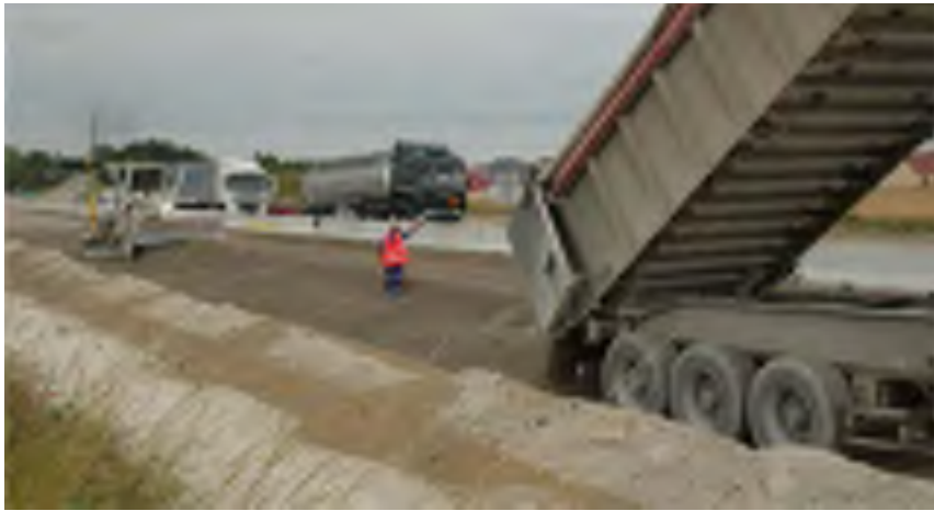
Figure 3 Laying of Recyvia® in the bypass of Troyes (France)
