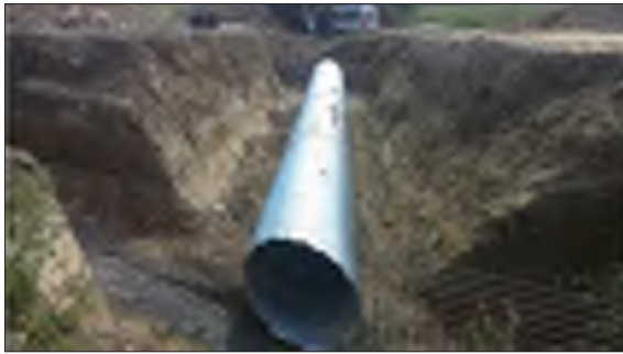
Figure 5 Assembly of pipe with coupling, backfilling and wall construction
