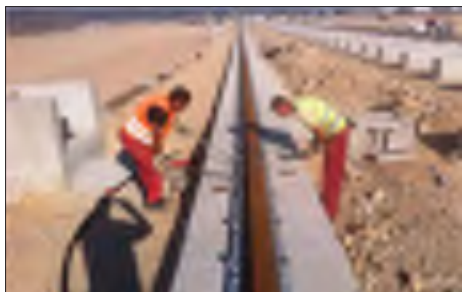
Figure 12 Phases of construction: alignment of the rails
