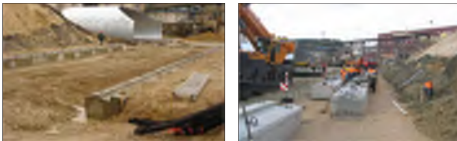
Figure 8 Supporting the soil-steel structures on piles
