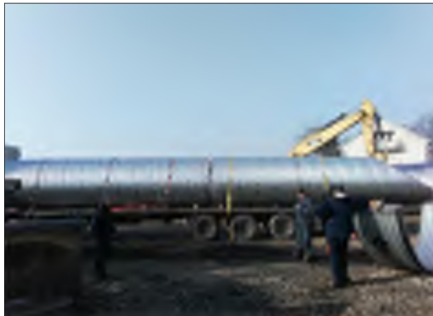
Figure 2 Transport of HelCor® spiral steel pipes
