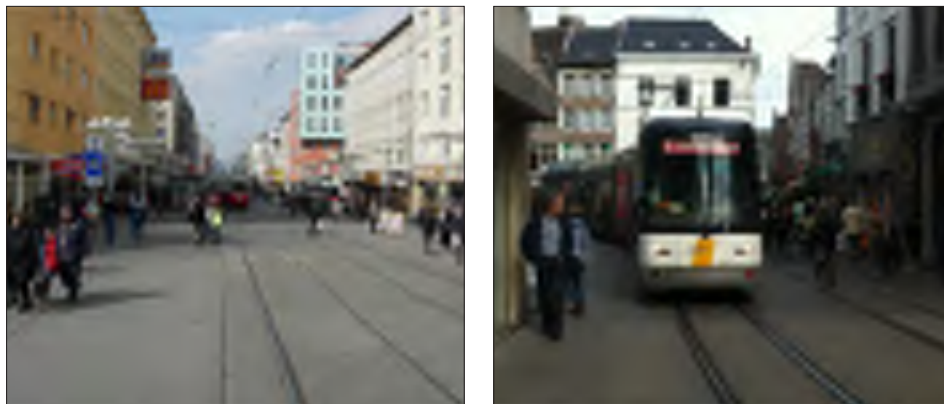
Figure 5 Road cross-section with tramway and pedestrian zone (Vienna, Austria & Gent, Belgium) as examples for a efficient and human-oriented design of transport infrastructure and public space.
