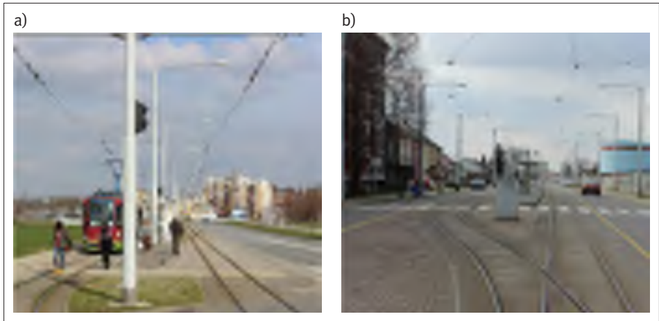
Figure 3 Tram stops: a) along the edge of the pavement, b) in the middle of pavement
