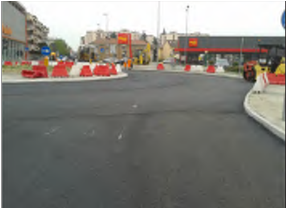
Figure 15 Wearing Course after compaction
