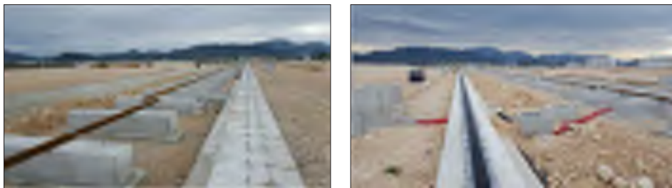
Figure 11 Phases of construction: integration of the elastic pads and rails
