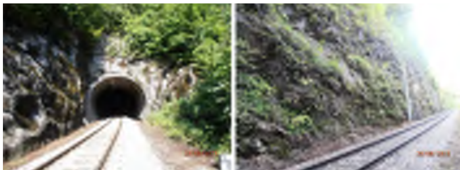
Figure 1 Entrance portal of tunnel Tičevo and the exit cutting
