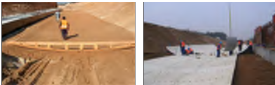
Figure 2 Classic closed-bottom foundation of soil-steel structures
