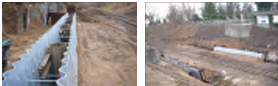
Figure 6 Supporting the soil-steel structures on piles
