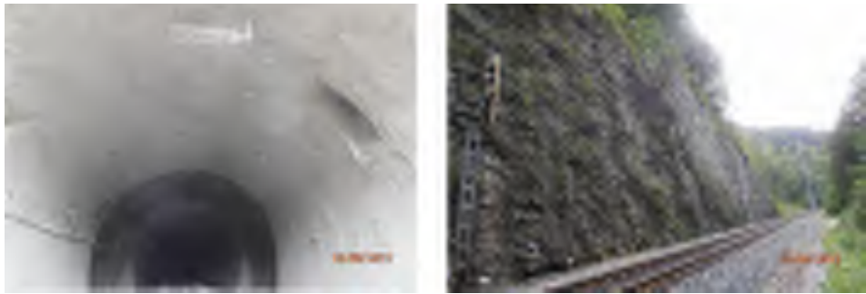
Figure 4 Reconstructed vault of the tunnel Tičevo and cutting exit of the tunnel
