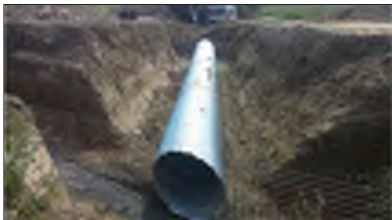
Figure 5 Assembly of pipe with coupling, backfilling and wall construction
