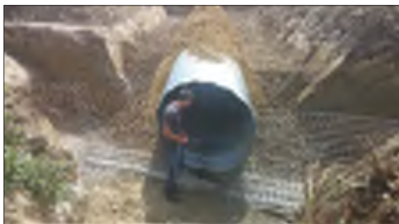
Figure 6 Both-sided backfilling with compaction and construction of walls
