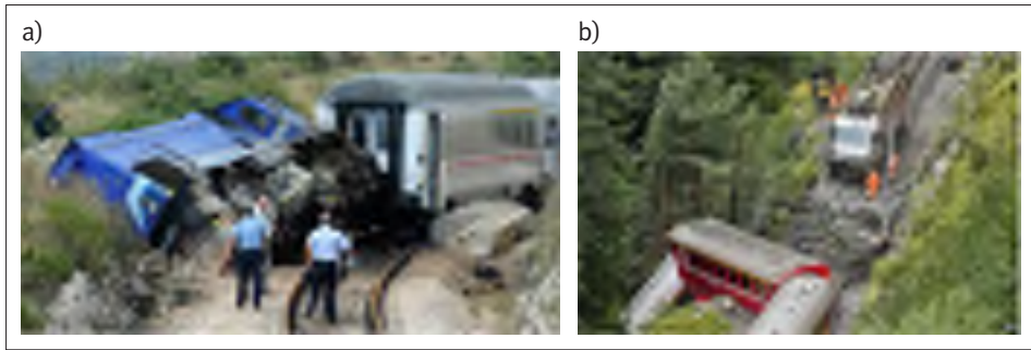
Figure 1 Recent railway failures: a) Rockfall on Zagreb-Split railway track in Croatia in 2014 [2]; b) Derailment of a Swiss train caused by a rainfall induced landslide, in 2014 near the Swiss Ski resort of St. Moritz [3]
