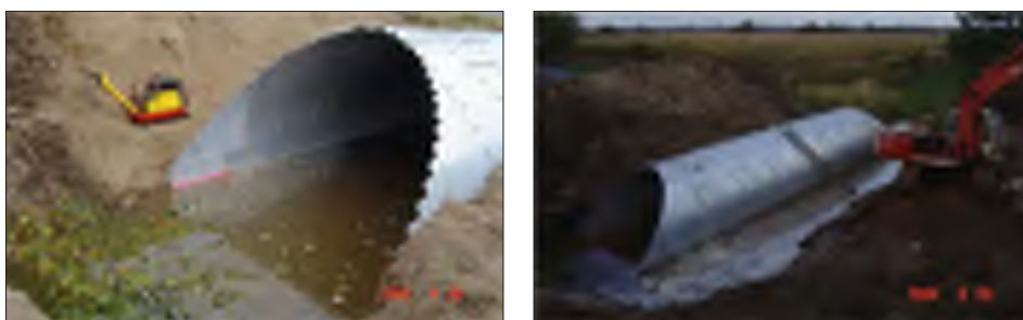
Figure 3 Initial phases of the construction of the structure in a watercourse
