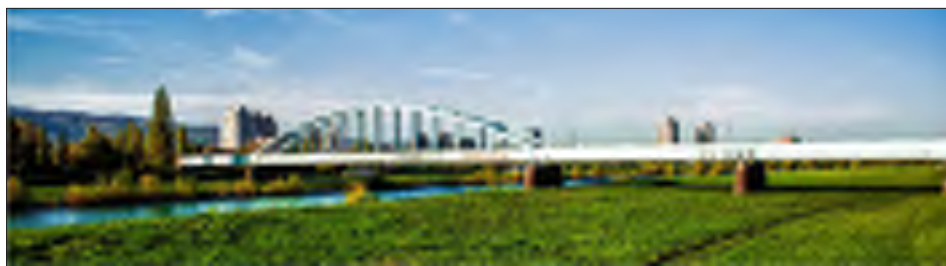
Figure 2 New bridge “Sava” before the strengthening
