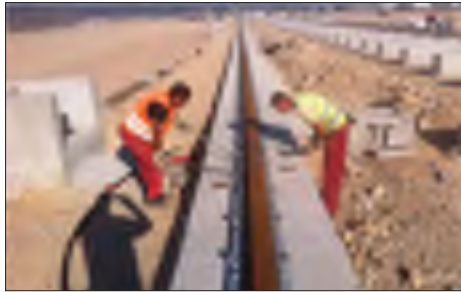
Figure 12 Phases of construction: alignment of the rails
