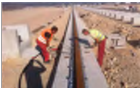
Figure 12 Phases of construction: alignment of the rails
