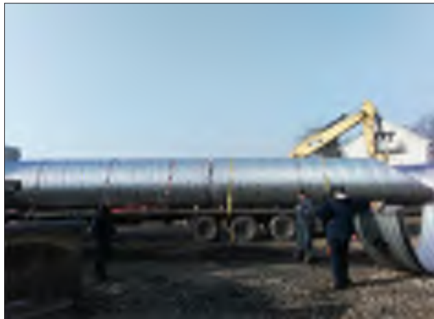
Figure 2 Transport of HelCor® spiral steel pipes
