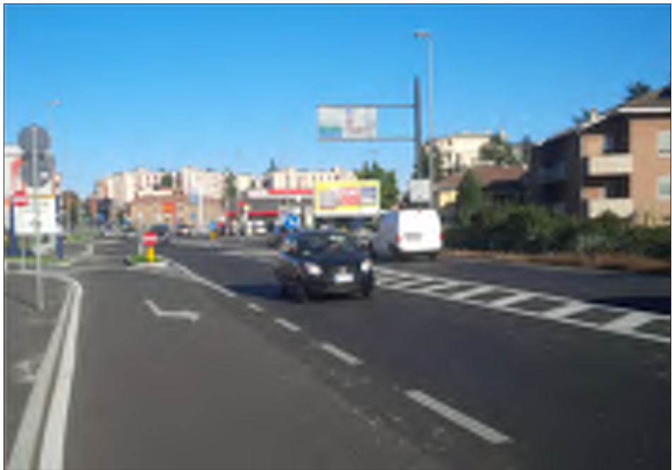
Figure 16 Corso Vercelli Street 3 months after construction
