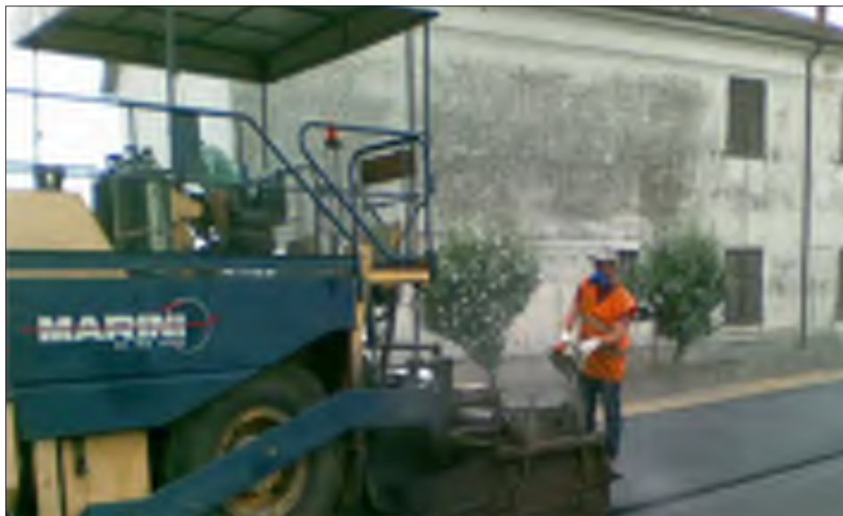
Figure 9 Laying of the wearing course
