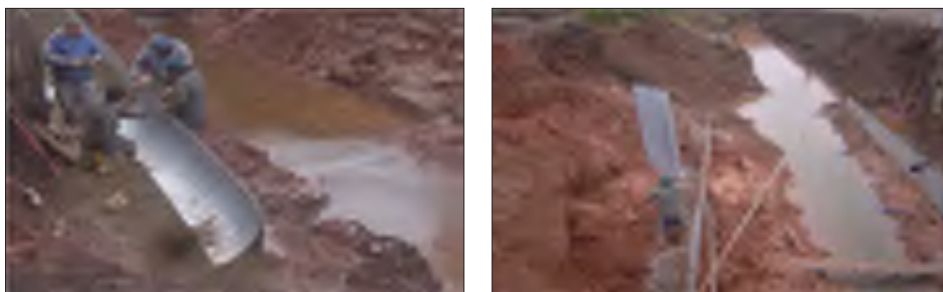
Figure 5 Corrugated sheet wall with a groin supported on the native soil
