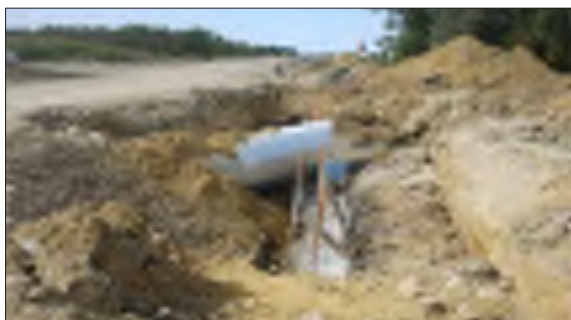
Figure 7 Culvert under traffic load during wall construction activities
