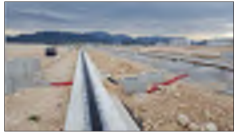
Figure 11 Phases of construction: integration of the elastic pads and rails
