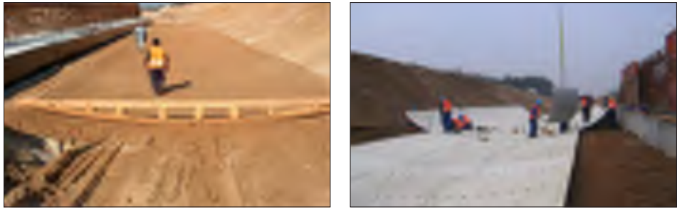
Figure 2 Classic closed-bottom foundation of soil-steel structures
