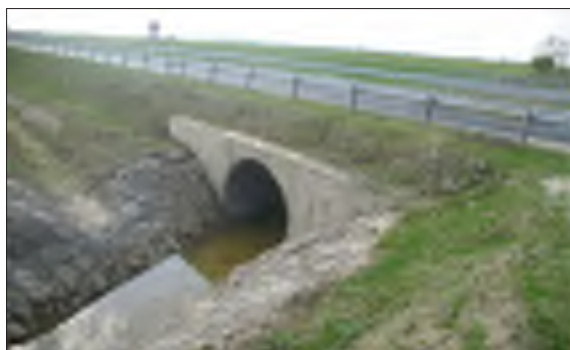
Figure 11 Completed culvert (CH 2000) in road bed during road use
