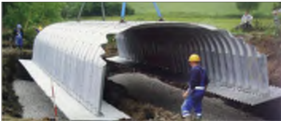
Figure 4 Erection of the corrugated steel structure with an attached support in the form of a flat sheet
