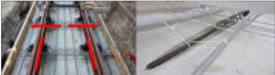
Figure 6 Position of strain gauges on reinforcement rod – 21-STT
