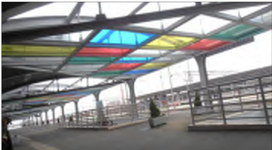
Figure 6 61 st platform of the railway station Slavovski Brod after reconstruction
