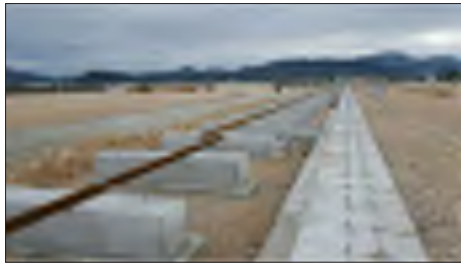
Figure 11 Phases of construction: integration of the elastic pads and rails
