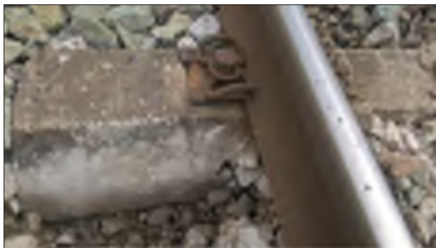
Figure 4 Replacement of ZEL.8 fastening with compatible fastening UTZ
