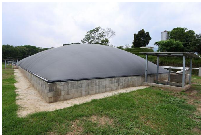
Slika 13. Lagunski digester (Anonymous 1, 2019).
