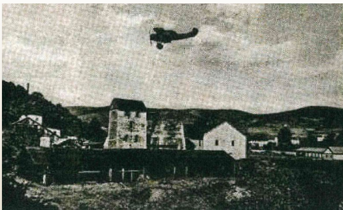
Blast furnace in Bešlinec / Visoka peč u Bešlincu, 1935 (from [4])
